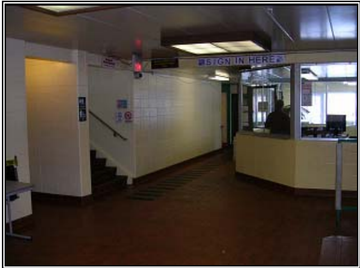
An outdated floor plan results in congestion and circulation issues in the building. Over - programming and program overlap exacerbate these problems, particularly at peak usage
